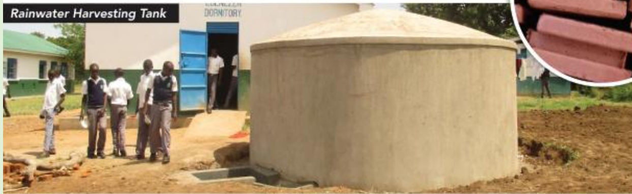
Underground Rainwater Harvesting Tank
